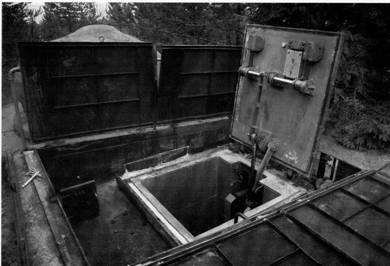
One of the entrances to the reserve fire command post (measuring station) on Hemso, built in 1973 - Photo By Dan McKenzie
